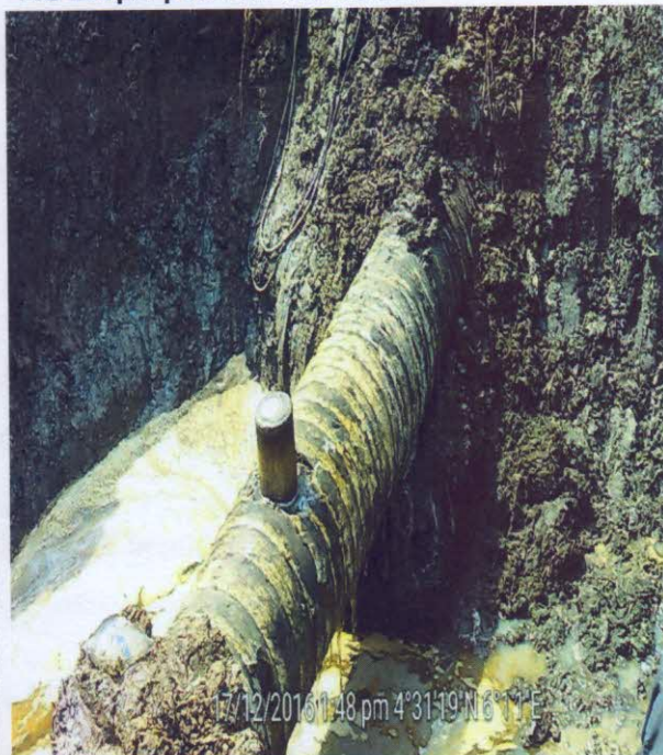
Repair of spill point (coning)
